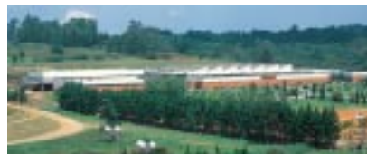
Suzano Plant (Brazil)
